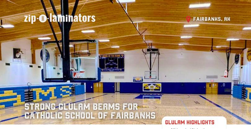
In 2021, multiple beam failures caused by heavy snowfall and wetter, heavier snow necessitated urgent structural reinforcement at the Catholic School of Fairbanks.
