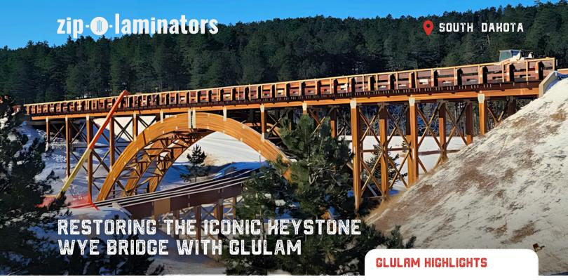
Near the majestic Mount Rushmore in South Dakota, the Keystone Wye Bridge has stood as an engineering marvel since 1968. After 50 years of service, an inspection revealed that while the glulam supports were in excellent condition, the concrete deck panels had deteriorated. Glulam decking was recommended as a long-lasting solution.
