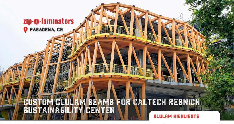
The Caltech Resnick Sustainability Center aimed to create a visually striking and structurally sound lattice-like curtain wall that would highlight the natural beauty of mass timber. The architectural and design team envisioned a glulam structure composed of beams, columns, and diagonal
