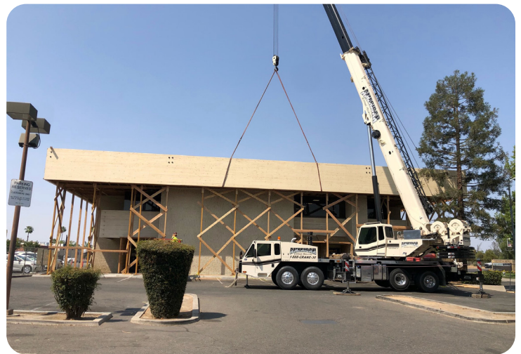
The Golden One beam in place
